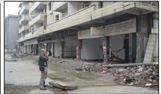
Destruction in Dujiangyan: several died leaping from this building in panic
