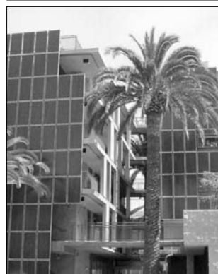
Photovoltaic panels used as architectural features on a Santa Monica studio apartment building
