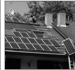
Photovoltaic and solar thermal panels being installed in Freiburg, Germany
